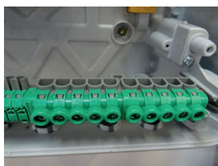
Earth terminal block: screw terminals
