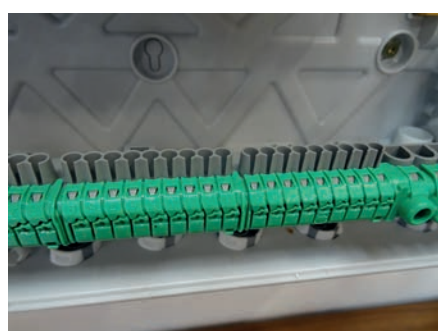
Earth terminal block: automatic connection
