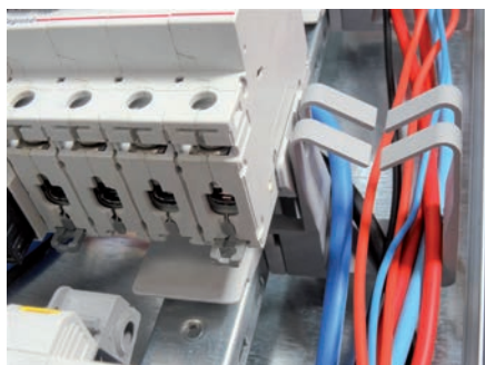
Holding vertical wiring in place
