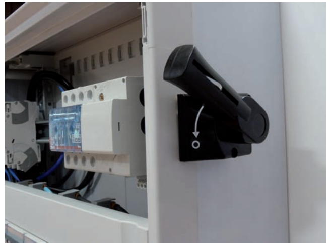
A template is provided with the side/front handle for drilling the side panel
