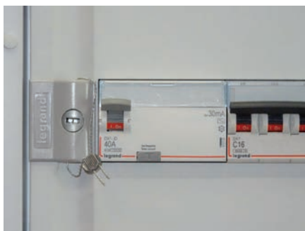
Sealing the faceplate, in locked position
