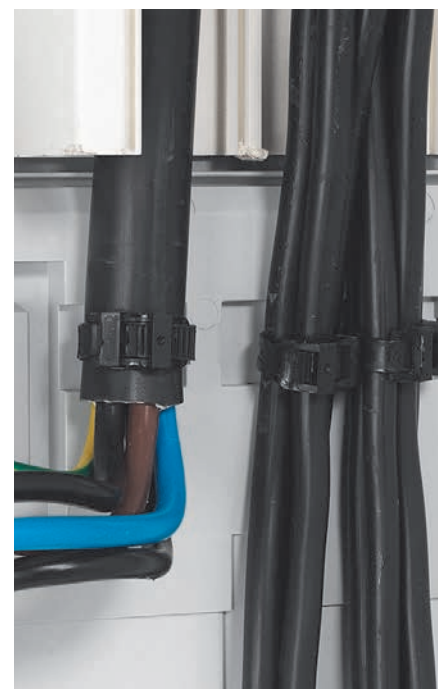
Anchoring the cables
