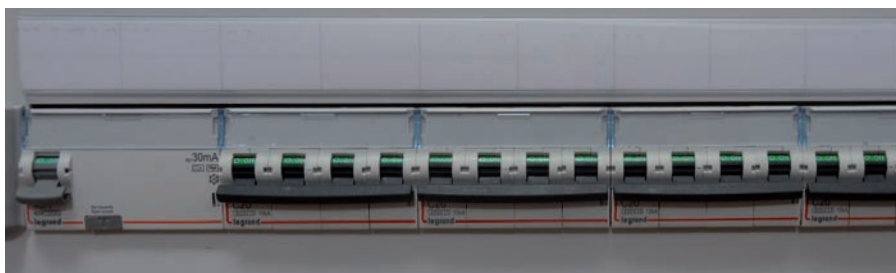
As well as the label-holders on all modular devices, a plastic marking strips Cat.No 3 397 55 (24 modules) or Cat.No 3 397 56 (36 modules) are available as accessories, supplied with the sets of labels
