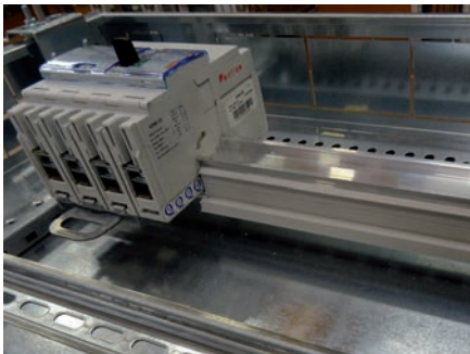
Mounting with a plate and the rail height spacer next to it
