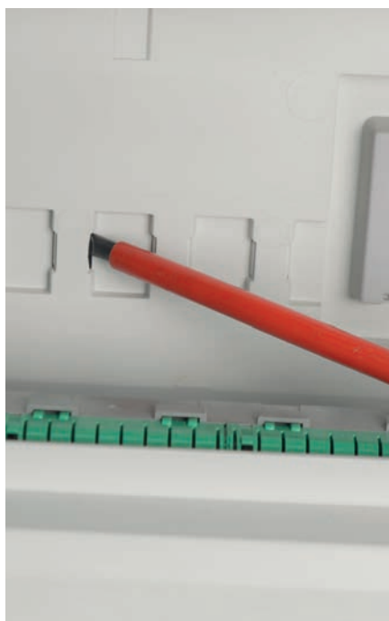
Knocking out the feedthroughs
