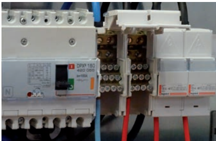
Modular single-pole distribution blocks: total isolation of poles in order to distribute up to 250 A (160 A max. in a XL 3 160 cabinet)
