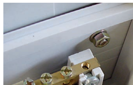
After refit the drilled and cut side panels, place the 4 screws and 4 M6 nuts in position, but do not tighten them fully.
