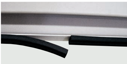
The seal must join up at the bottom of the door
