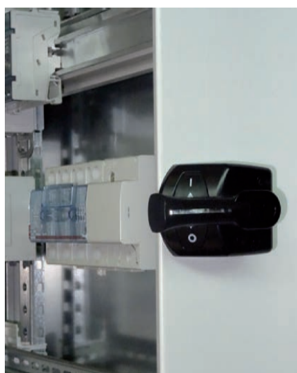
The handle is mounted directly on the cabinet side panel.
