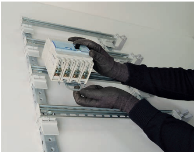
Mounting the assembly on the chassis by removing the plastic rail support
