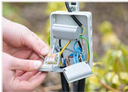
Connecting a bollard light
