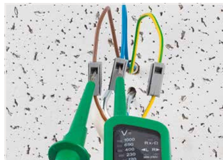
Testing via separate test ports.
